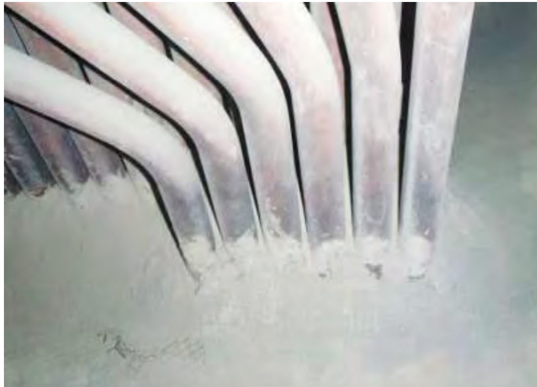
Original ISOMEMBRANE® Installation in 1994
